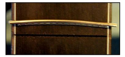
The "tang" of the fret wire (the portion of the fret that is forced into the fret slot of the fingerboard) must be removed from the fret at each end. In the above photo, a close look reveals that the tang has been clipped and filed or otherwise
